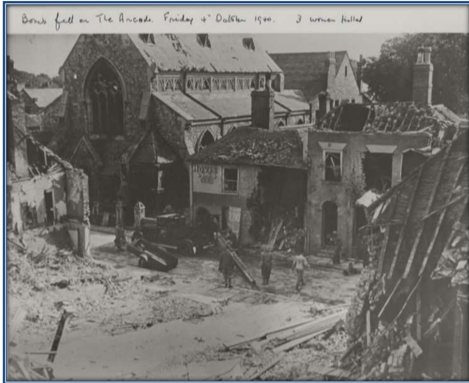
Bomb Damage 4 th October 1940
